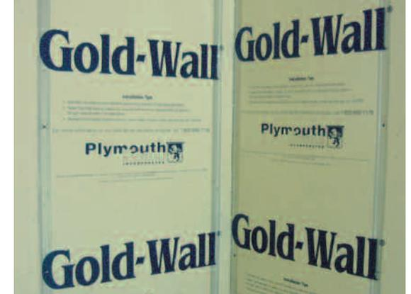
Minor in the field trimming offers the ability to easily float inside drywall corners.
