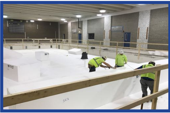
Boldt Workers Installing The Durafill Blocks
