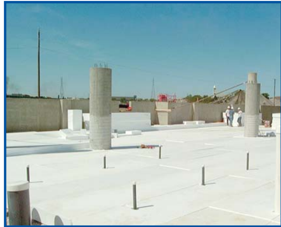
Cuts easily around plumbing and other structural elements.
