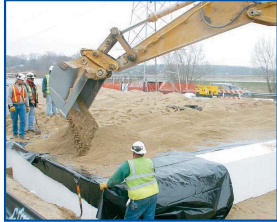
Fill weight reduced by up to 130 lbs. per cubic foot when replacing standard dirt and gravel.
